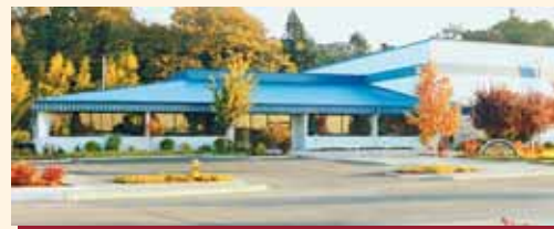
Columbia/Okura, LLC headquarters, Vancouver, WA USA
